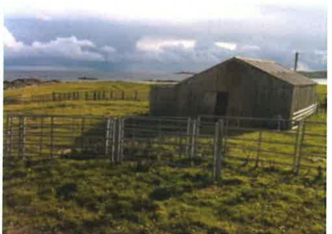
Existing agricultural shed with cattle pens on site of a previous mart (to be demolished).
