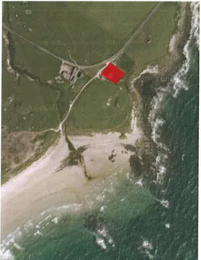
Aerial view of site with Soroby Beach to south and Crossapol Farm to west.
